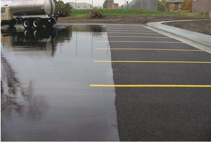
Non-porous asphalt vs porous asphalt
